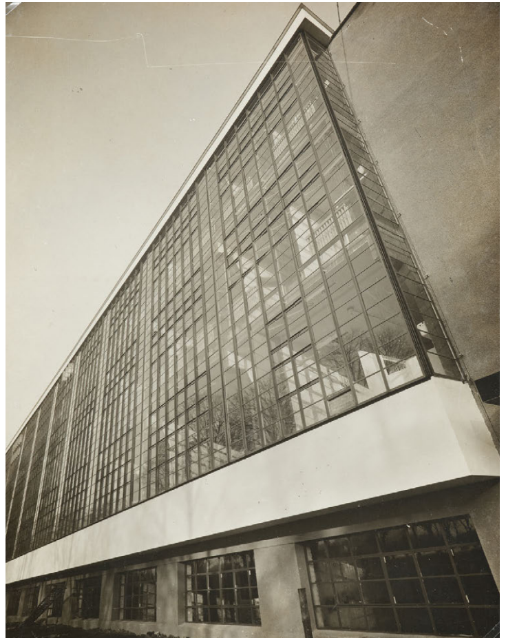
Lucia Moholy, Bauhaus Workshop Building from below
